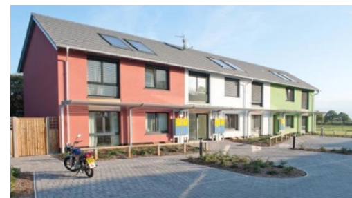
Wimbish Passivhaus certified. (Source: Hastoe Housing Association)
