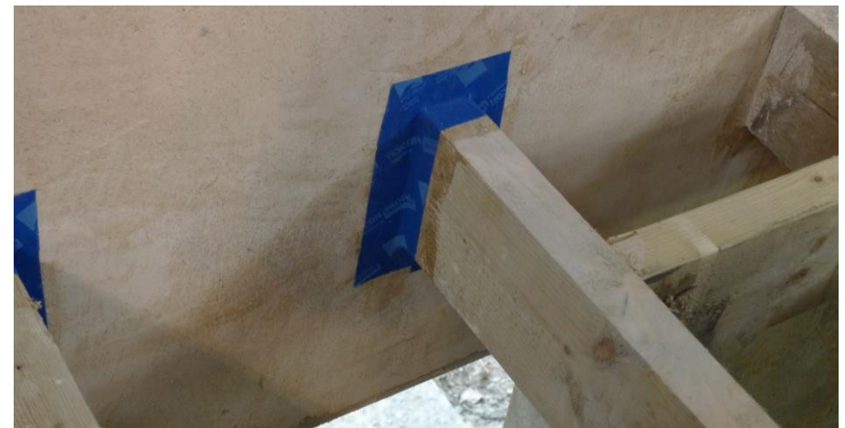
Applying airtightness tape to joist ends is a common measure required to achieve good airtightness in existing buildings. Large gaps may need filling with mortar first, and remember to apply a suitable primer. (Source: Ecomerchant)
