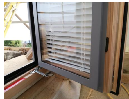
Replacement triple glazed windows (Source: Internorm)
