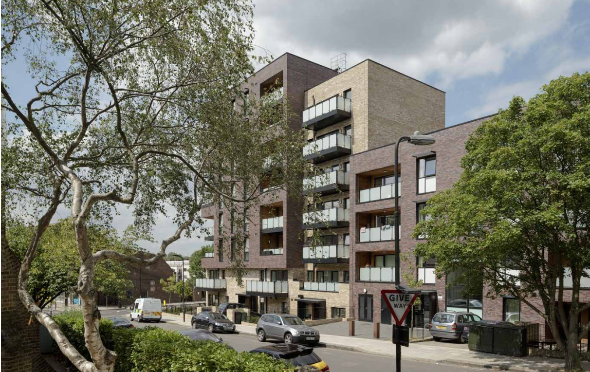
View from the southeast showing the stepped façade
