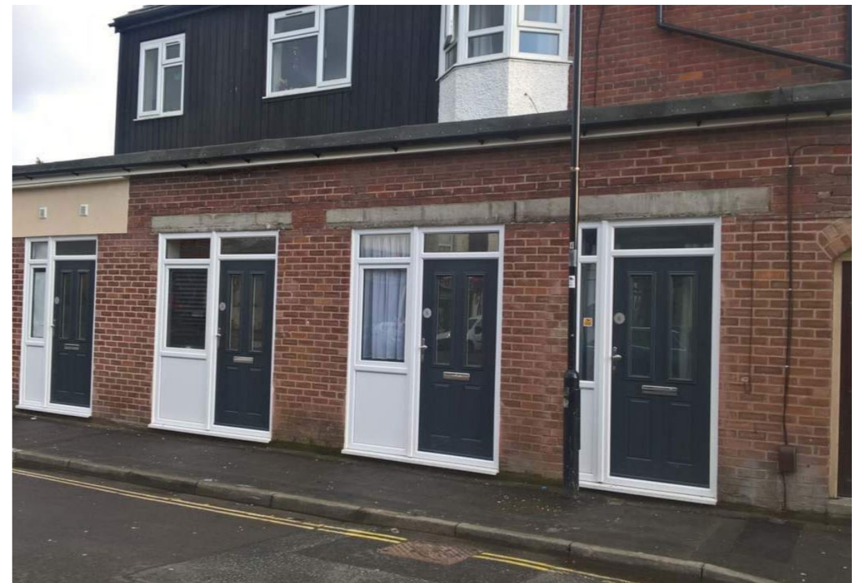
Shirley Road, Southampton – after: converted into six studios
