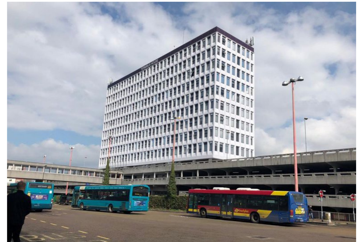
Terminus House, Harlow
